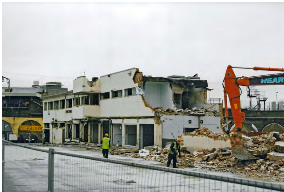
Above: Two weeks later, and significant progress had been made. 24 January 2005. See also photo on page 28.
