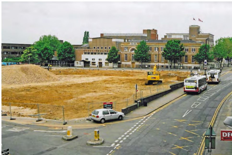
Below: The view from Chelmsford Railway Station bridge after the demolition had been completed.
