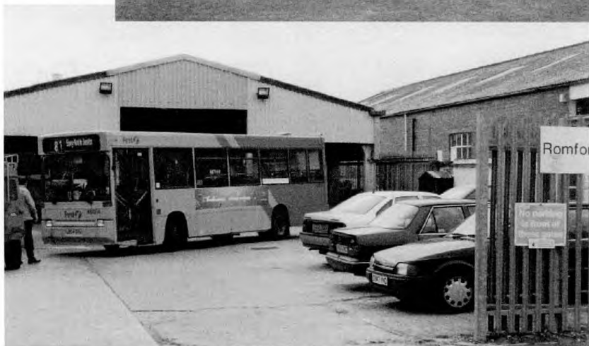
Romford (RD): "Sorry - Not In Service" - at least as a First Essex depot. The premises and operations were transferred to First London in September. Dart 46804 manoeuvres on the last day (17th).
