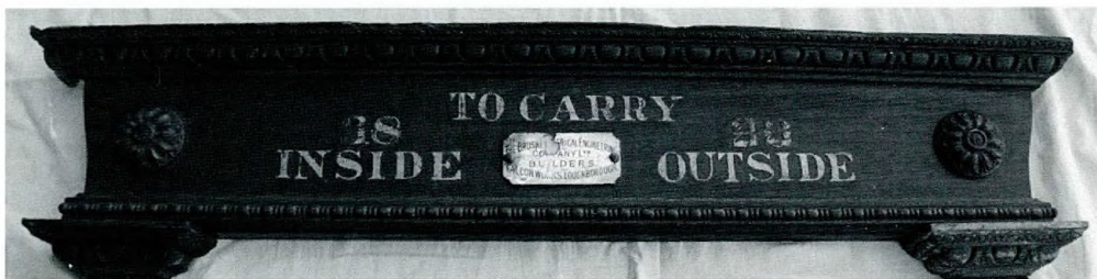
A close up of the door lintel.
