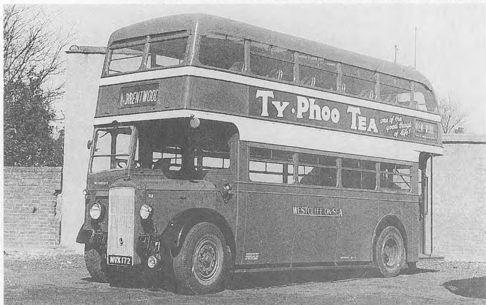
Part of City's large post-War double-deck intake, 1949 Daimler CVD6/Roberts D2 is seen in Brentwood depot after gaining full Westcliff (green) livery, complete with silver grille. As fleet number 1217, NVX172 was withdrawn by ENOC in 1962. (Alan B Cross)
