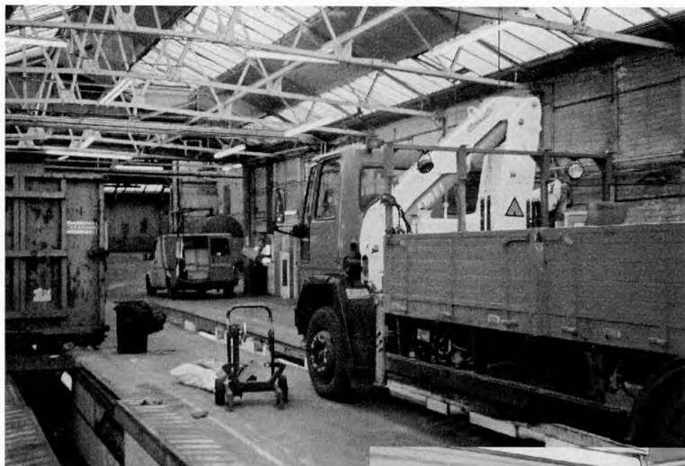
3 April: Maintenance bays with Chelmsford's Ford Cargo truck 90235 (E157 BTL) and Transit van 90233 (L631 VAE) clearing the site.
