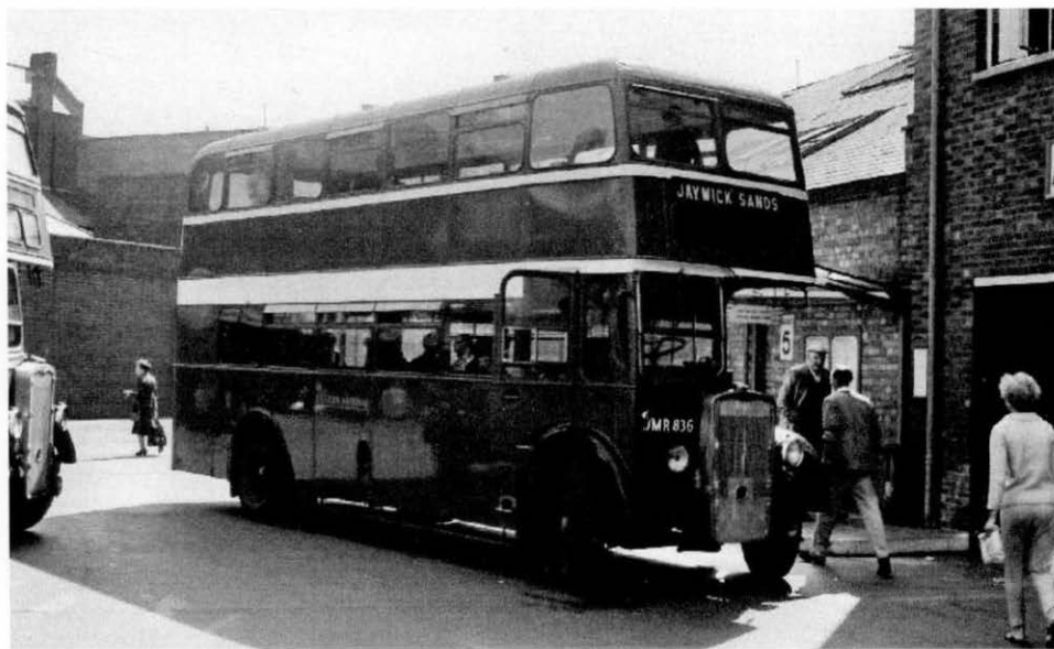
A busy scene in Clacton Bus Station, with ex-Wilts & Dorset 1051 (DMR 836) about to leave for Jaywick. Two W&D peculiarities are evident: the rain louvers over the rebuilt opening windows, and the three-piece indicator with single-track number box (albeit with via and number boxes painted out).
