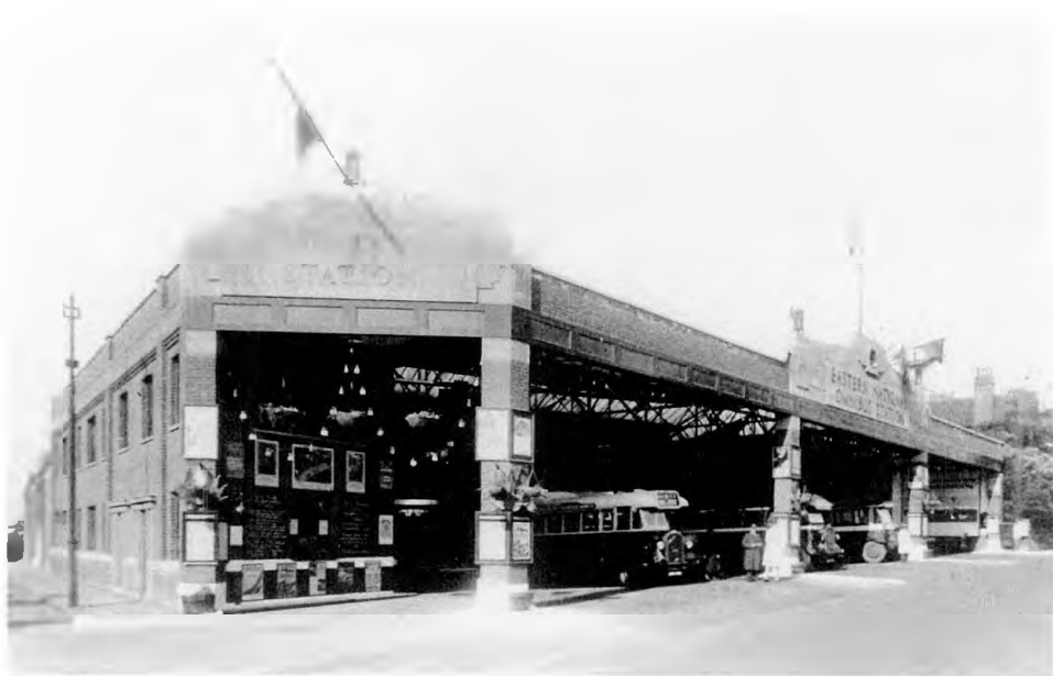
above: Bus Station (2), c1931: Counting House, Enquiry Office/house demolished and new covered bus station constructed, extending northwards to Fairfield Road. 'EASTERN NATIONAL OMNIBUS STATION' in relief on the facade. Three Dennis Lancets waiting. Floral baskets and flags in abundance. Was this opening day?
