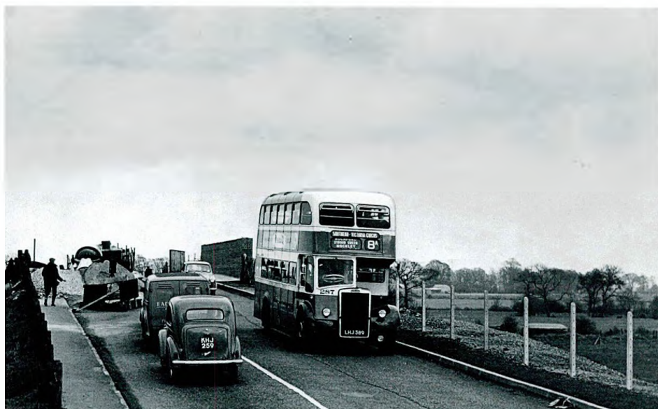
Then and now (2) One bridge that does not present an obstacle to deckers is Warners Bridge near Southend Airport. Our "then" view from 1956 shows new Leyland PD2/Massey lowbridge 287, passing roadworks on the bridge in connection with the electrification of the Southend Victoria line ...
