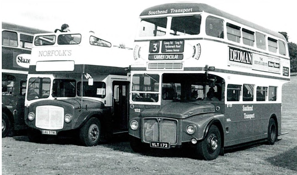
Above: STRM11 - 102 (VLT 172), RM172. Right from earliest days, RM172 became the ST 'showbus' RM, as was the fad in the 1980s in London, with chromed headlamp surrounds, full depth heater grille, brake cooling grilles, LT fleetnumbers (including red bonnet flap) and chrome front wheelnut guard rings (which were only fitted for rally appearances). 102 (VLT 172) was the only RM repainted a second time into my original livery design.
