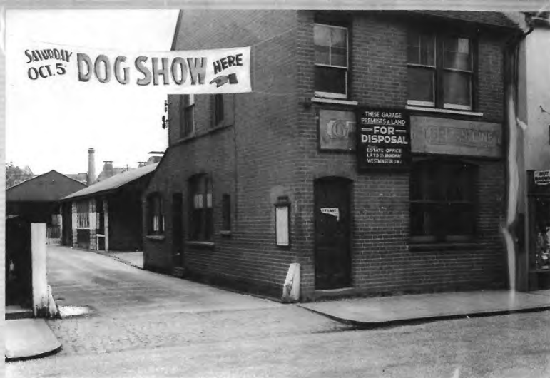
The London Transport waiting-room (formerly London General, and prior to that owned by Acme Coach Co.), on the site of the present Erentex cleaners in South Street. Taken in Sept. 1936, after closure of the ex-Acme garage, seen in the background.
